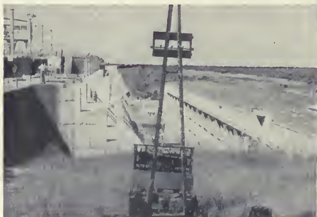
RIO NEGRO dam and power plant in Uruguay, an outstanding example of durable concrete construction and modern engineering.
